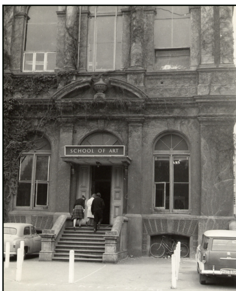
Entrance to the South Australian School of Art, Exhibition Building, North Terrace, Adelaide. Photograph by Allan Sierp, Head of SASA 1961 to 1963.
